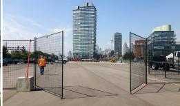
Modu-Loc fence systems include pedestrian and vehicle access gates. Our gates can be placed anywhere in the fence line, allowing for effective control.
