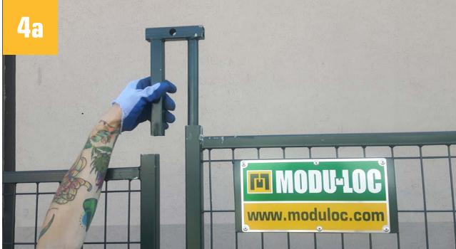
**IF USING CAPS:** Now you're ready to finalize the fence set-up by installing the caps. All the caps also consist of one square and one round peg. These need to be installed in the same fashion that the bases were laid out: round pegs line up with round pegs and square with square. Insert the cap into the top of the panel, and slide the cap in completely.
