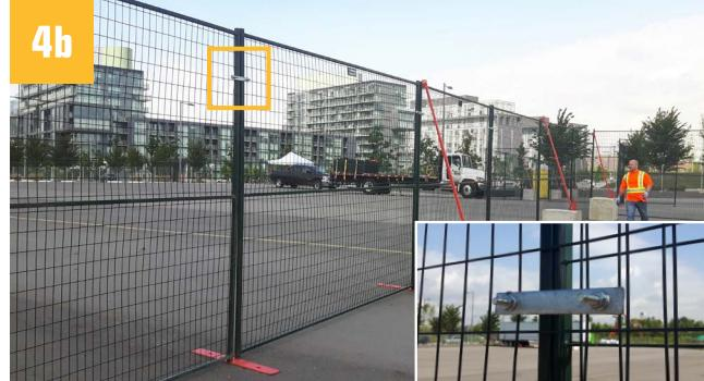
**IF USING U-BOLTS:** Now you're ready to finalize the fence set-up by installing the u-bolts. U-bolts are installed at approximately 6 ft high, connecting two panels. The bolts should be securely fastened and face into the site.
