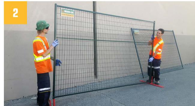
With a partner, begin assembling the fence panels onto the bases. Insert the square peg into the panel first, then drag the panel back to the previously installed base and place it on the round peg.
