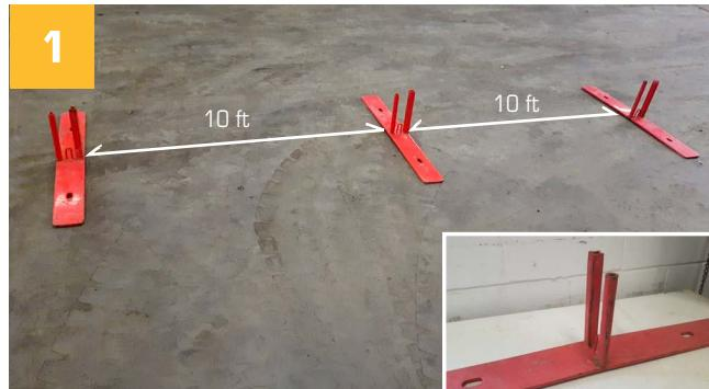
All Modu-Loc fence bases consist of one square and one round peg. Lay out fence bases 10 ft apart with all of the round pegs facing the direction you will build your fence.
