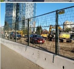
Modu-Loc Fence Rentals offers superior installation systems that adapt to the most demanding conditions, including roadside applications. Modu-Loc fence can be mounted on concrete or jersey barriers, providing additional security and privacy for roadside installations.
